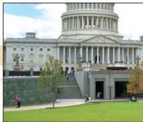
The southern entrance to the Capitol Visitor Center in Washington, DC
